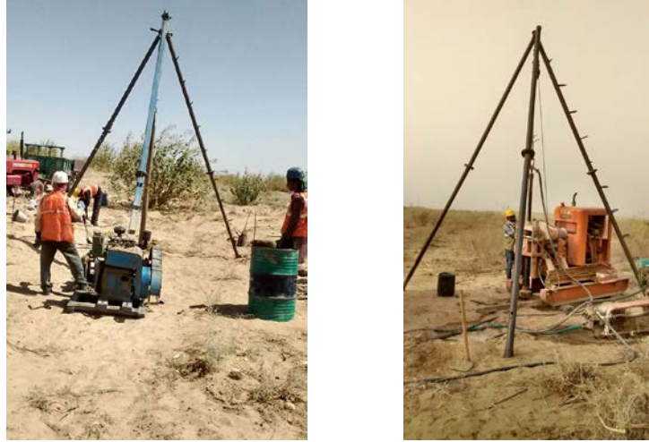
Fig. 2. Boreholes in progress. Photo on left illustrates soil boring in progress using mechanized shell and auger. Photo on right illustrates rock coring being done using hydraulic rotary rig
